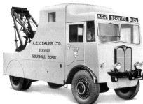
Owned by A.C.V. Sales Ltd., at all its Service Depots, the 4-wheel drive "Matador," fitted with a manually operated crane and incorporating a winch on the rear of the cab, is a highly useful breakdown vehicle.
